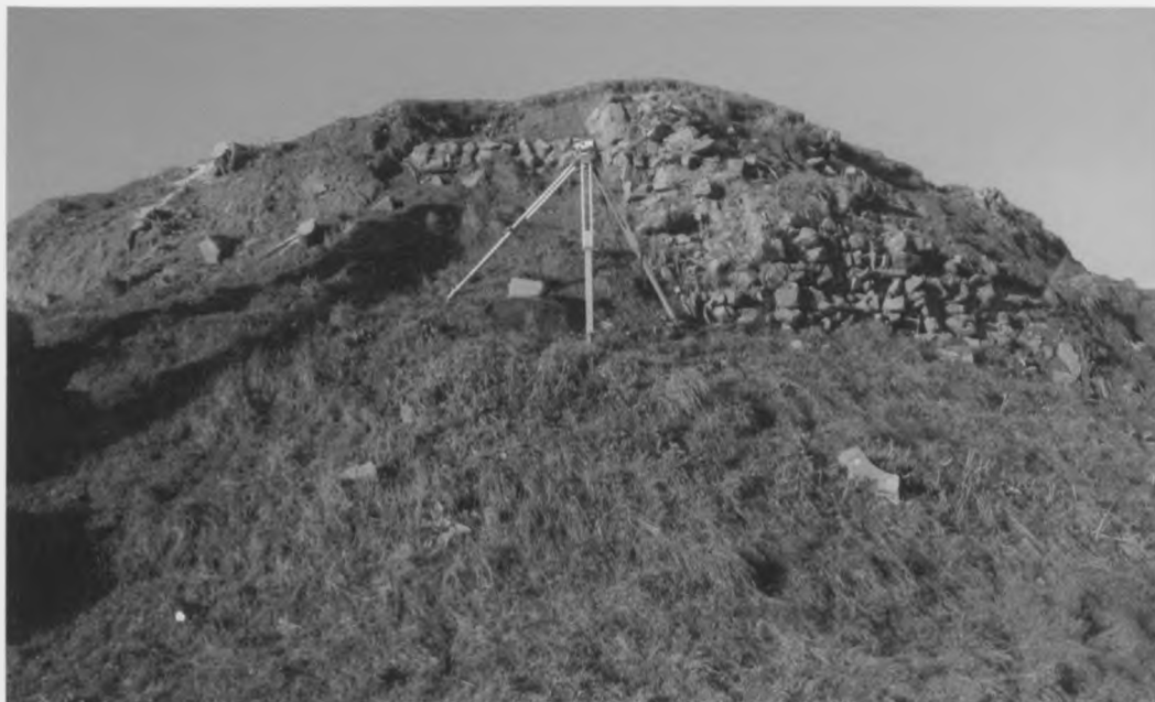
Plate 5: Caerwent motte . Roman masonry revealed by erosion of southern half of mound. By courtesy of Cadw. Crown Copyright.
