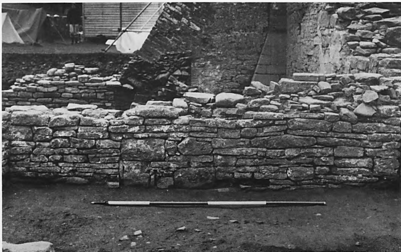
Plate 12 East wall of phase III and IV chapels after removal of plaster; viewed from the west.
