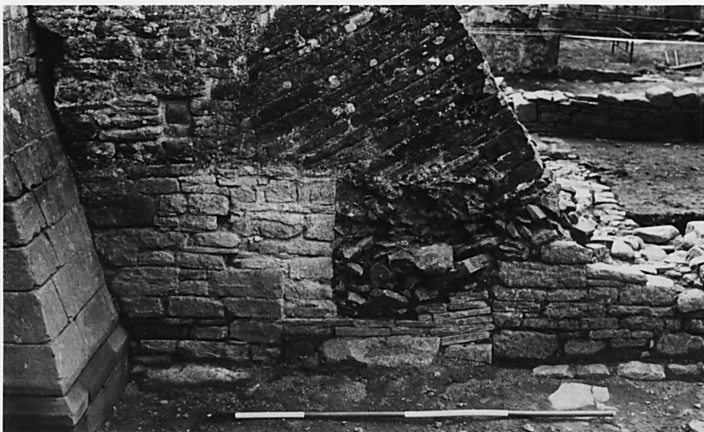
Plate 13 Buttresses in the south-east corner of the phase II chapel. (viewed from left to right) Phase I external pilaster buttress: late medieval double offset buttress: 19th-century temporary buttress: phase II chapel wall.
