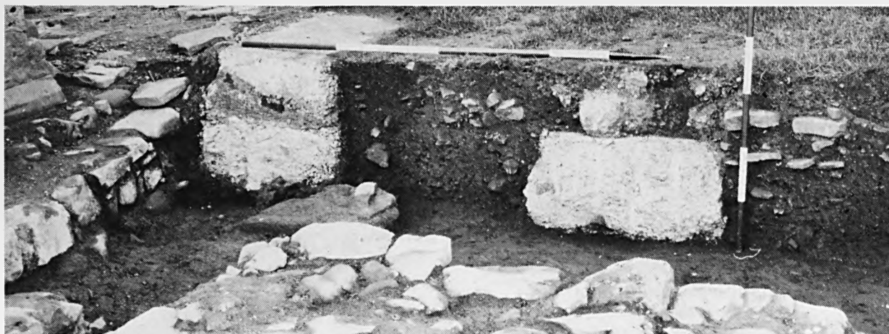
Plate 18. The 1930's concrete rafts under the crossing tower.
