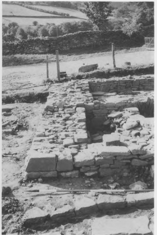
Plate 22. South wall of Phase II 'Infirmary' showing external batter.
