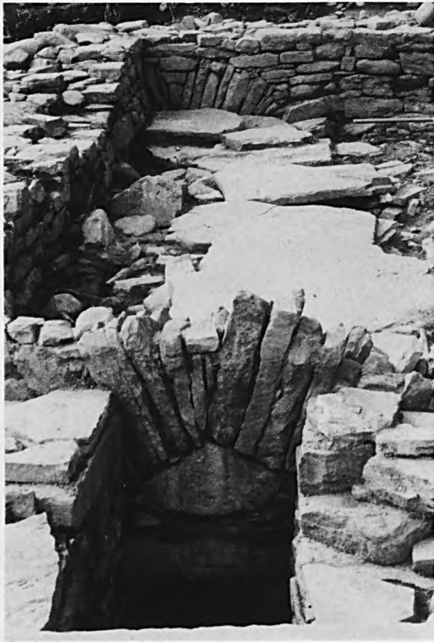
Plate 23. Sewer vaulting in wall 401.
