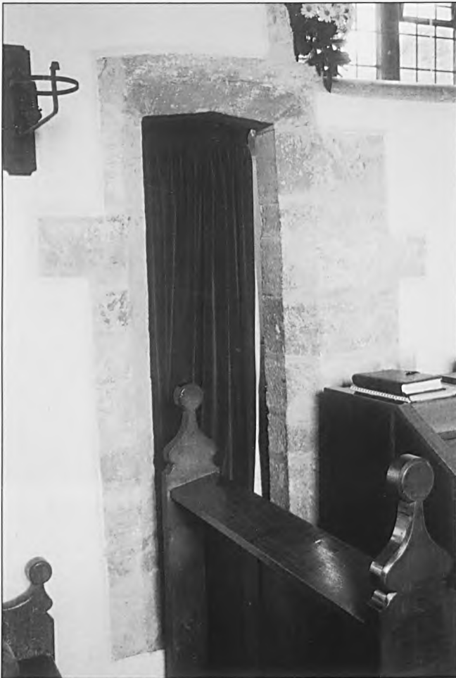
Fig. 10: the entrance to the late medieval rood loft stair at Tredunnoch church. (Copyright: National Museum of Wales)
