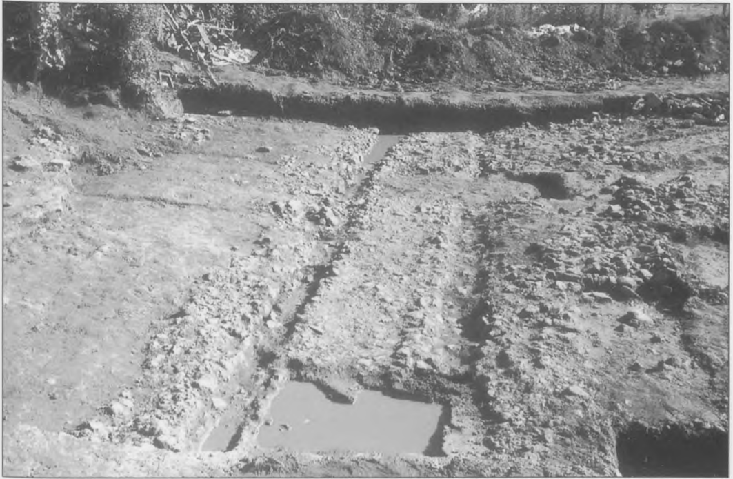
Plate 1: The road, from the south after heavy rain.
