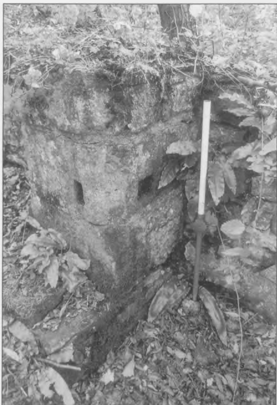
Fig. 18: mortises on the south pier of the chancel arch of Kemeys Inferior. (Copyright: National Museum of Wales).
