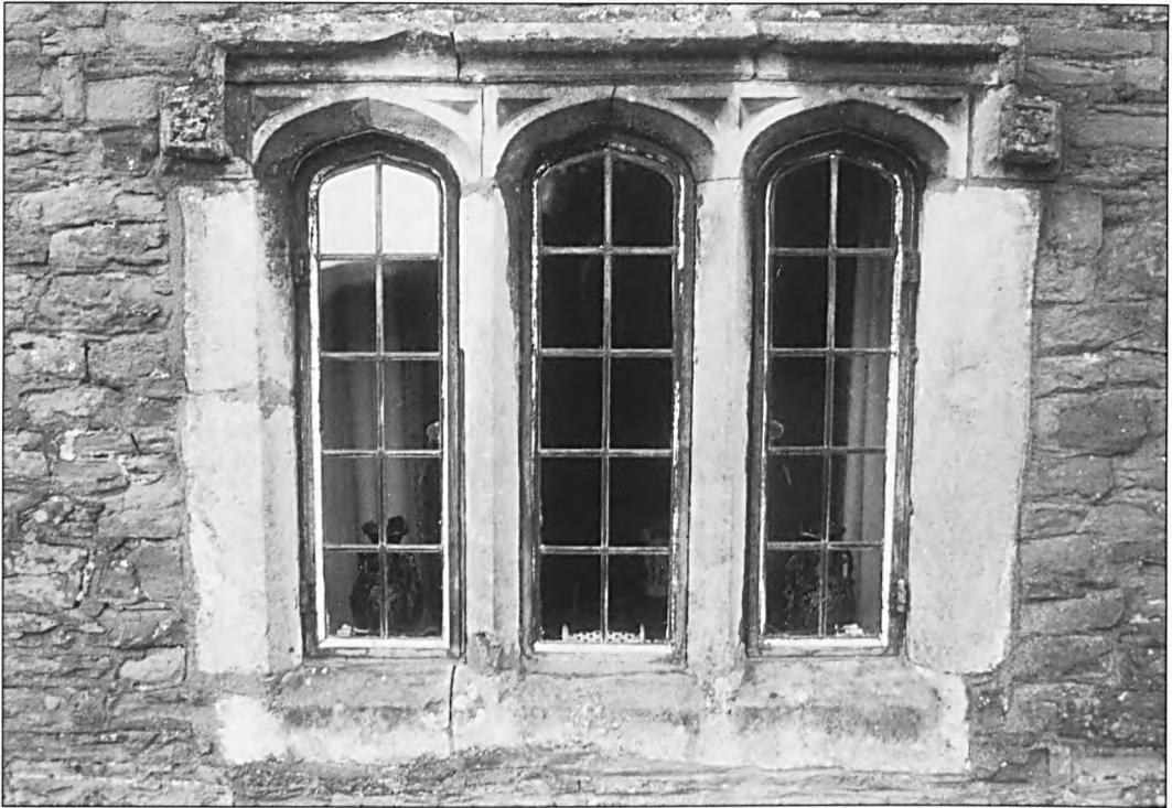
Fig. 16a: surviving tracery from the south wall of the nave of Kemeys Inferior Church, now reset in a south-west facing wall of Kemeys House. (Copyright: National Museum of Wales).
