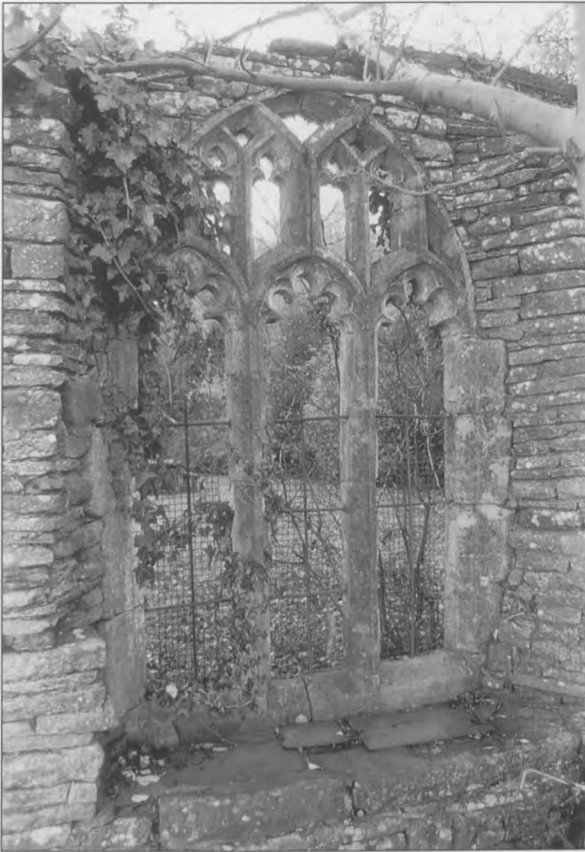
Fig. 16b: surviving tracery from the east end of the chancel, reset in the grounds of Kemeys House. (Copyright: National Museum of Wales).
