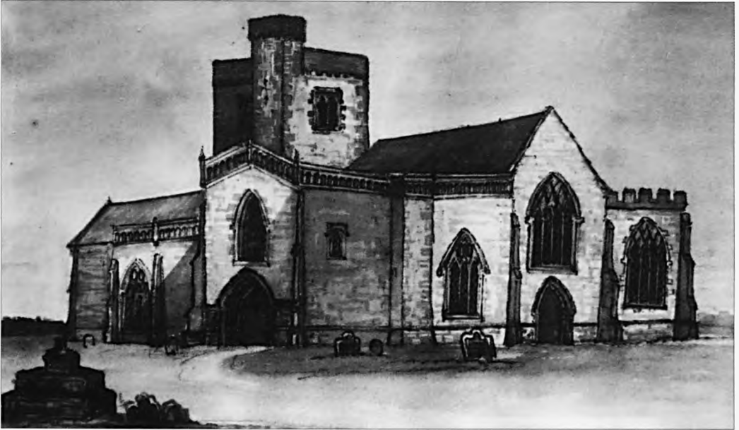
Plate 22. Magor: Church of St Mary (Gwentia III, 15). External stonework restored in 1861–1868.
