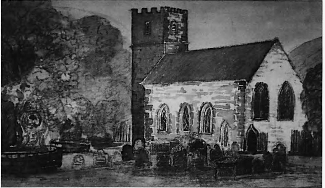
Plate 1. Aberystroth: Old church (Gwentia I, 2). Rebuilt in 1854–56, demolished c.1967.
