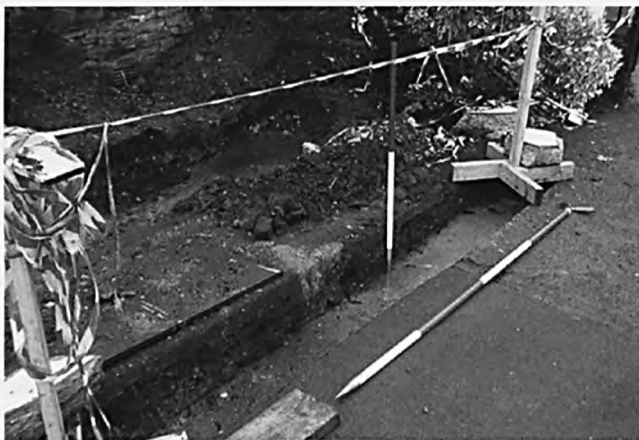
Figs 2, 3: The excavated foundation trenches with poured concrete footings on 14 January 2008.
