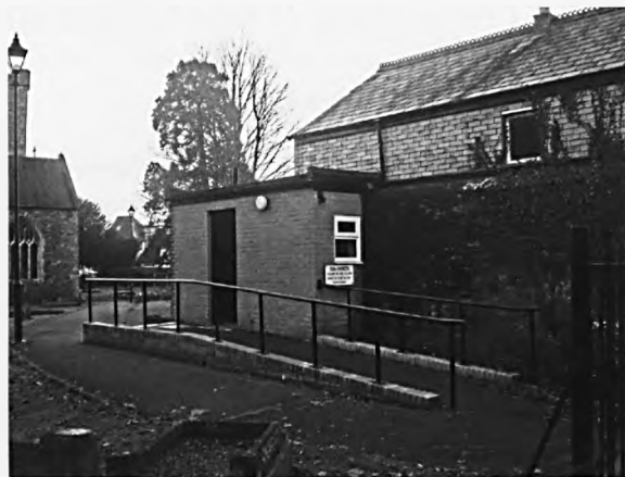
Fig 1: The completed church hall access ramp.
