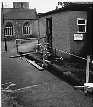
Figs 2, 3: The excavated foundation trenches with poured concrete footings on 14 January 2008.
