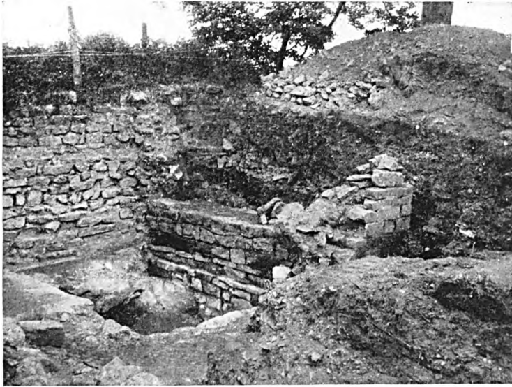
FIG. 5 The south corner-turret, 1909. The semicircular raft belonging to the rebuilt fortress-wall appears within the turret-area. Note the dressed courses above the offset in the fortress-wall within the turret; the tothing to the side-wall of the turret; and the ashlar front wall of the turret, with its false jointing. The fortress-wall, inner face, beyond is rough. ( From the Archaeologia Cambrensis, 1913, by courtesy of the Editor. )
