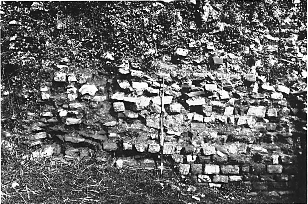
FIG. 3 The fortress-wall at the south corner, 1909. The joint between the original construction and the rebuilding can be seen about 2½ ft. to the left of the pole.
